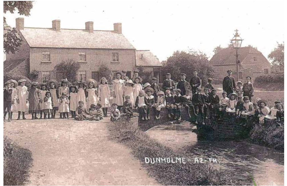
Fig 9: View from footpath along the beck looking towards the village green (1907)
