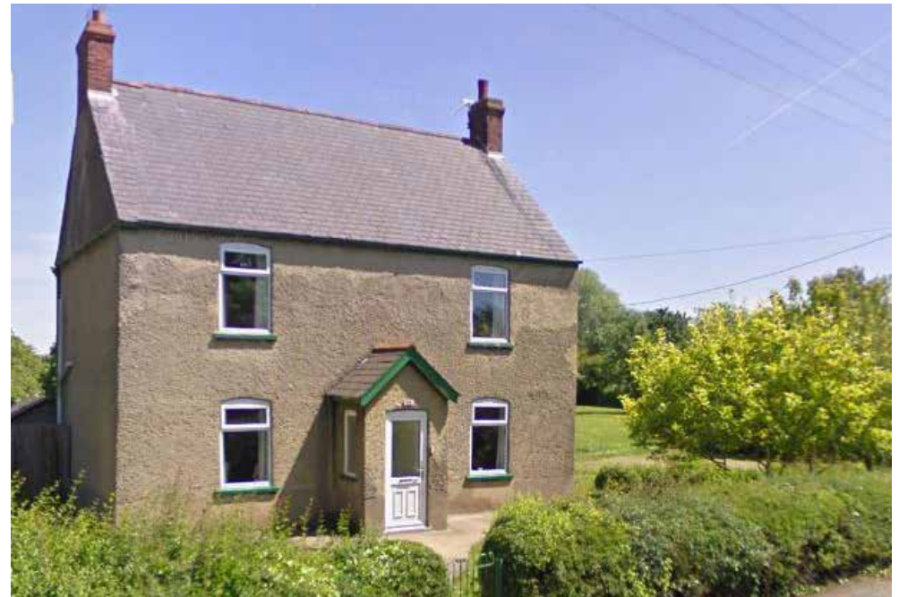
Fig 55: 28 Ryland Road has a symmetrical facade with a central entrance door and end chimney stacks
