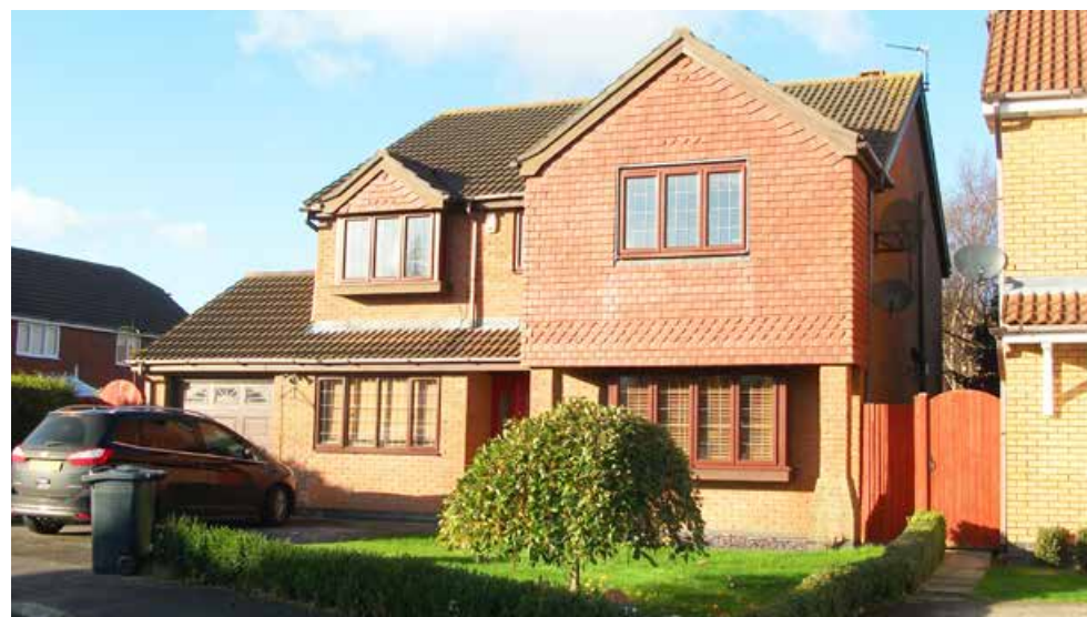
Fig 100: Hanging tiles are just one form of a particularly wide-ranging spread of external finishes that can be seen across Oak View, Wentworth Drive, and Beech Close
