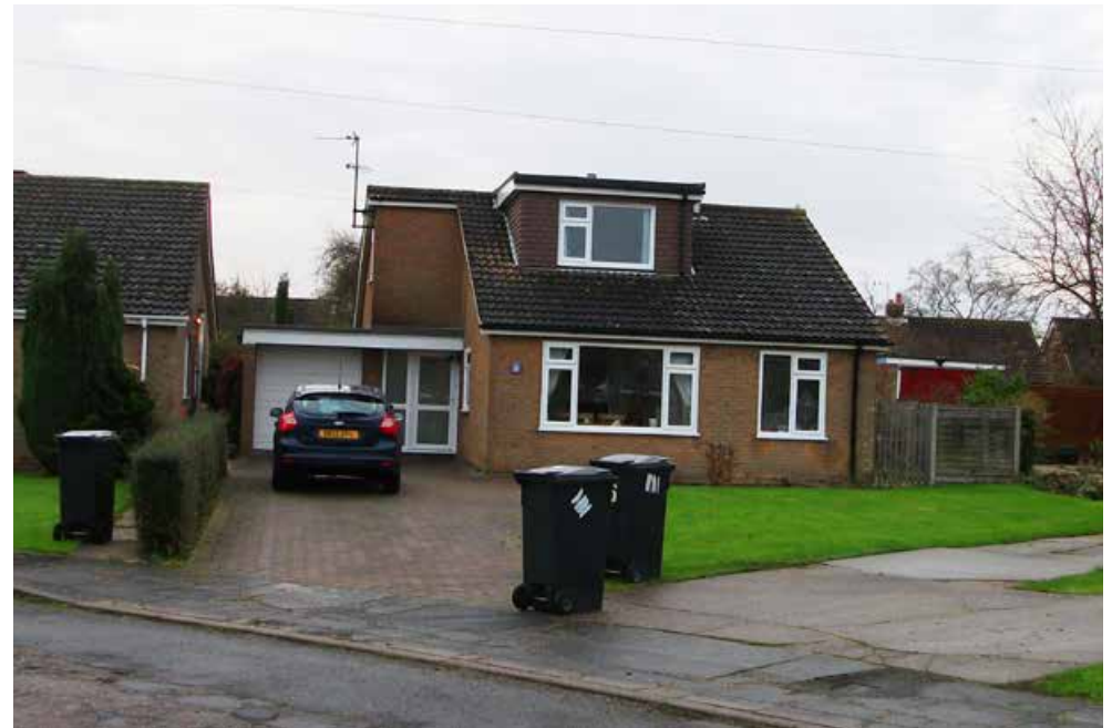
Fig 73: Numerous properties have been modified to accommodate rooms in the roofspace
