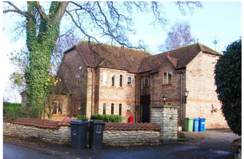
Fig 143: 7 Holmes Lane takes up a prominent position behind St Chad's Church
