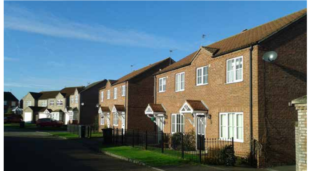
Fig 170: Semi-detached properties along Nusery Close, which create an uncharacteristically consistent building line
