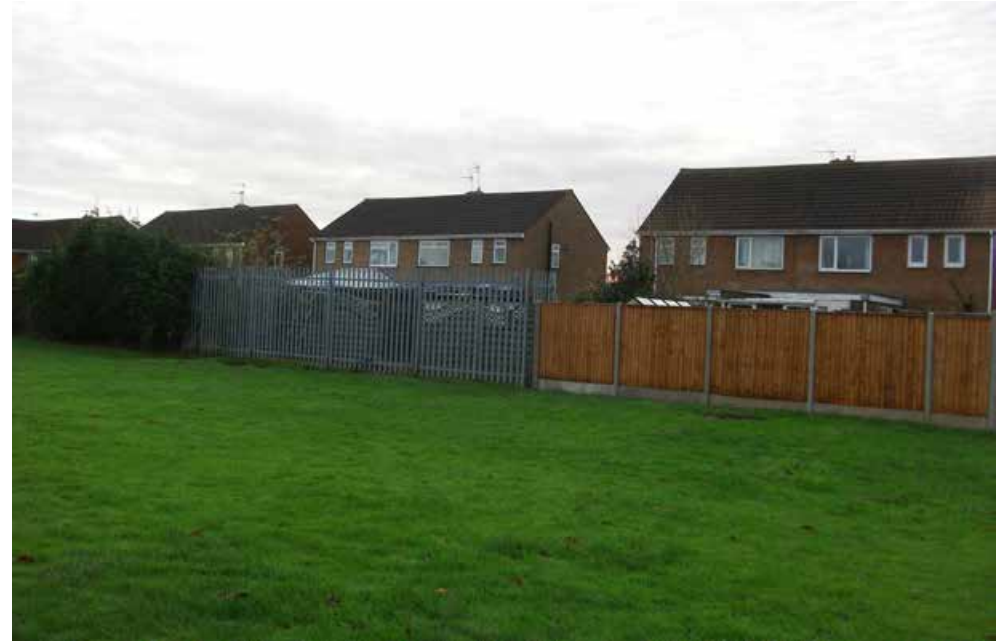
Fig 66: The southern and eastern edges of the recreation area enclosed by a mixture of differing boundary solutions, which undermine the aesthetic quality of the space
