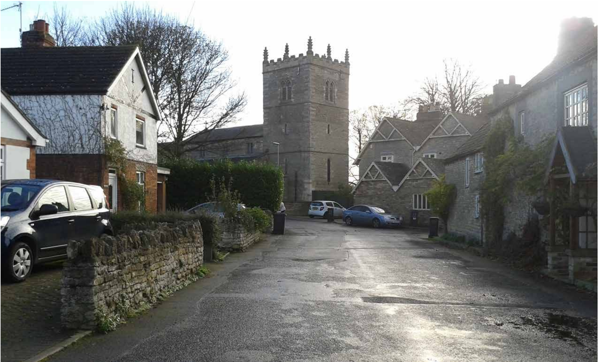
Fig 144: St Chad's Church and the vicarage building form a distinct group within the historic core of Dunholme
