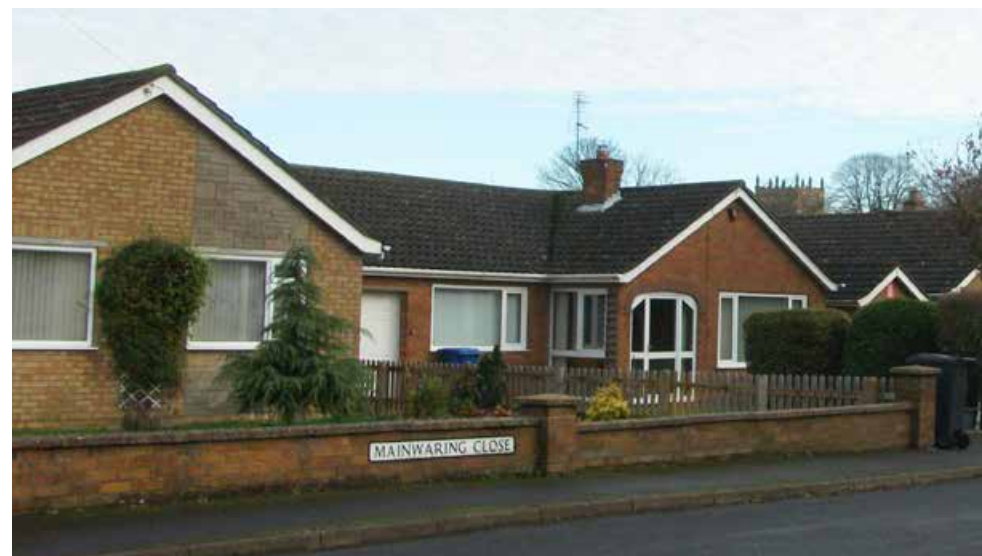
Fig 123: The single-storey form of the Mainwaring Close properties allows for views towards St Chad's.
