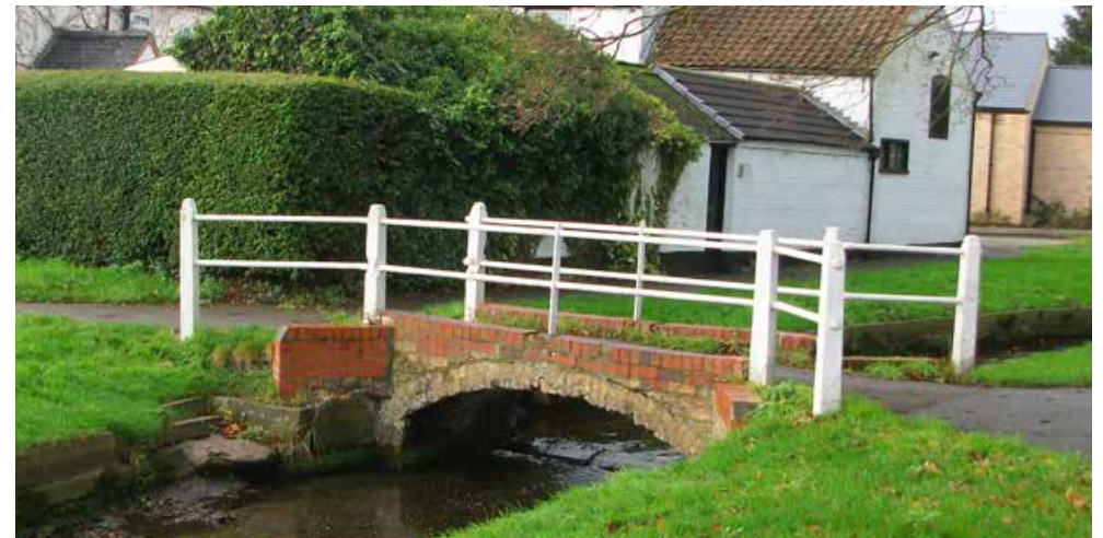
Fig 16: The brick bridge is a small-scale but highly endearing structure in the village centre
