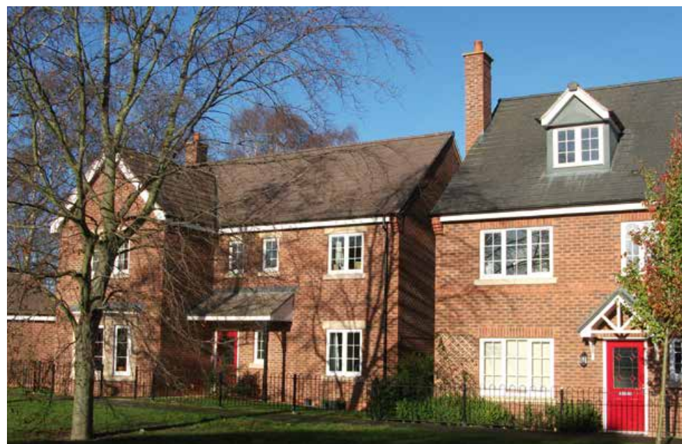
Fig 96: Properties within Four Seasons Close have well-proportioned facades
