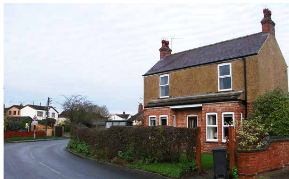
Fig 124: 4 Ryland Road is one of the most striking buildings within Character Area G
